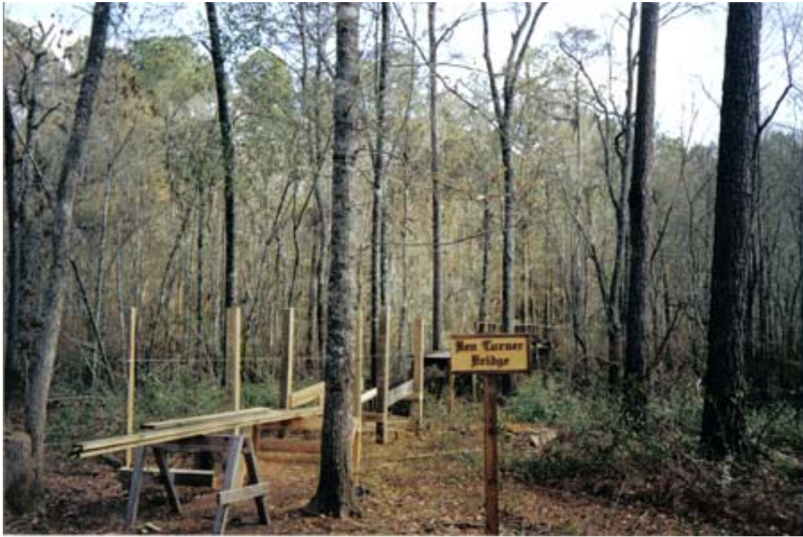
Ben Turner Bridge Under Repair
