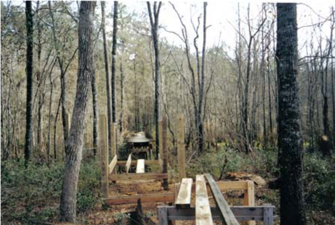
Ben Turner Bridge Under Repair
