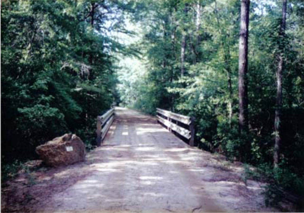
Bridge crossing creek between dining hall and lake
